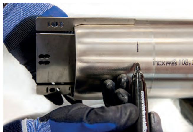
Figure 29 - Marking the Insertion Depth Using a Marker Ø 76 mm - Ø 88 mm - Ø 108 mm
