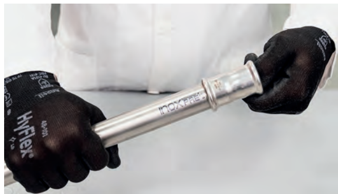
Figure 36 – Inserting pipe into the press fitting
