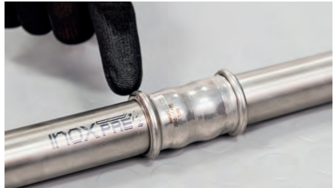
Figure 38 - Checking the press connection
