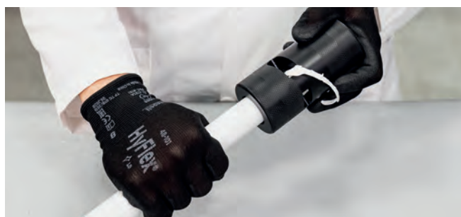
Figure 31 - Stripping [steelPRES PP coated]
